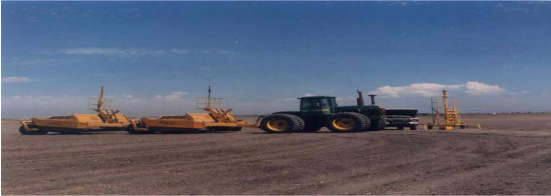
Figure1. Mechanized Laser Beam Field leveling
