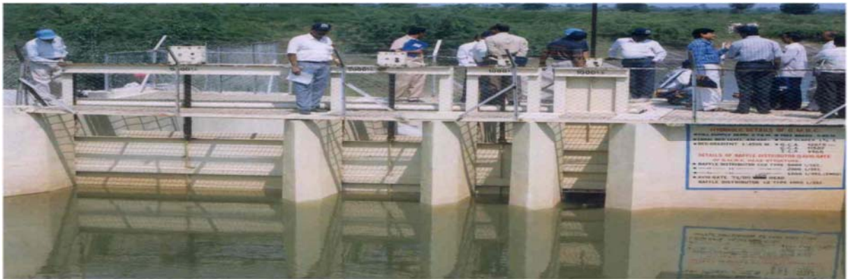
Figure3. Canal Automation , Cross Regulators ,Majalgaon Irrigation Project ,India.
